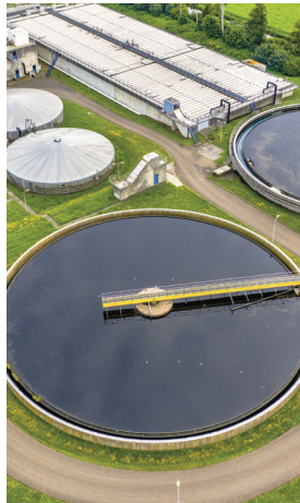
Water Treatment and Pressurization
